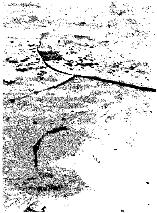
Fig. 2. Wide cracks with bowl-like rising of edges.
